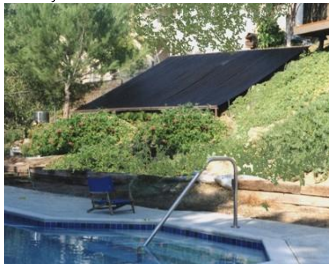
The black panels near the pool side are metallic heat exchangers that absorb solar energy efficiently, and this cost-saving energy to heat the pool.
