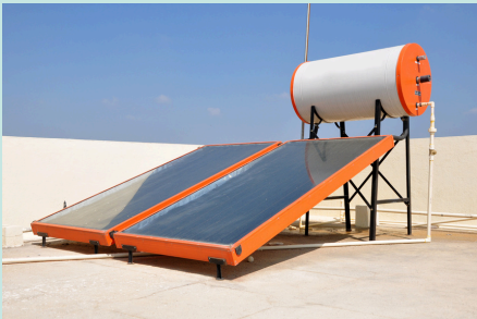
Solar water heaters.
