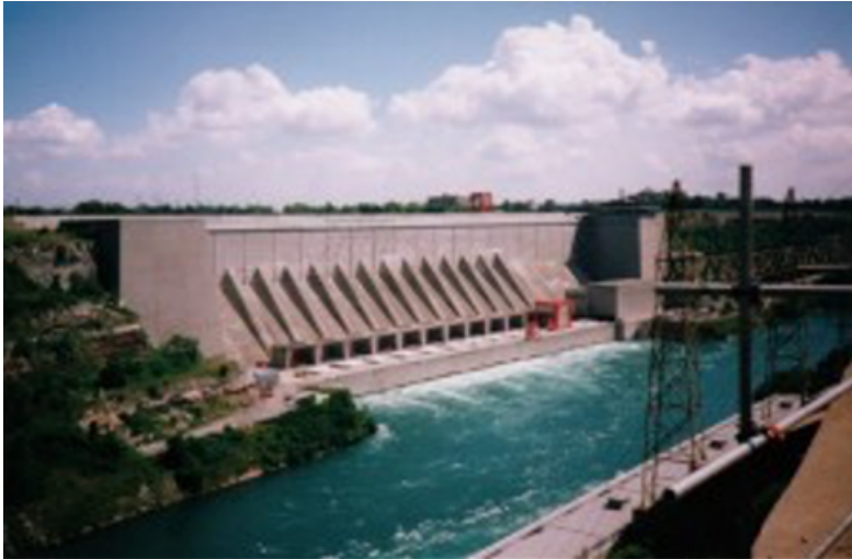
Hydroelectric facility in Ontario, Canada. Photo Courtesy of Shutterstock.
