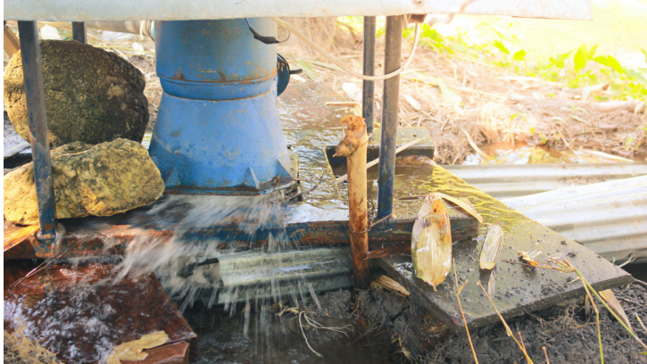
Example of a micro hydro system that can be used in rural communities.
