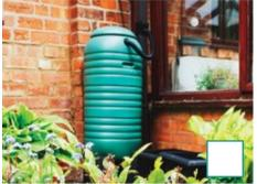
Put a 'V' if the rain barrel has a way to direct water at least 2 metres away from the house when it is full (e.g. with overflow pipes or connections to other rain barrels) or if water flow is blocked to the rain barrel when it is full and sent back into the downspout using a diverter (as shown in the photo).
