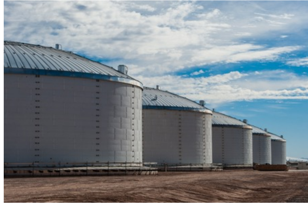
Molten salt storage tanks at the Solana Generating Station in Arizona, USA
