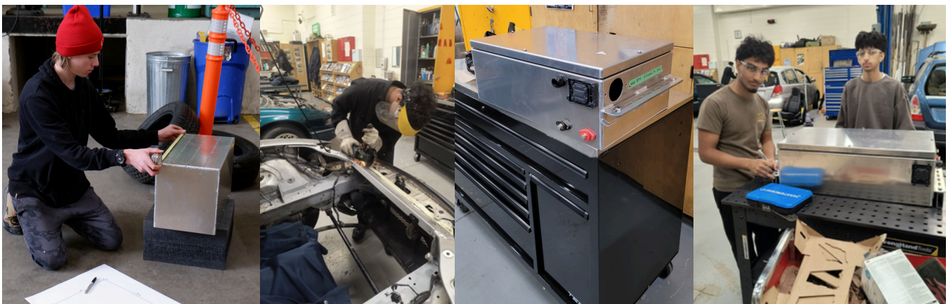
Students at both high schools taking measurements, welding, and working on the battery boxes in preparation for installation.
