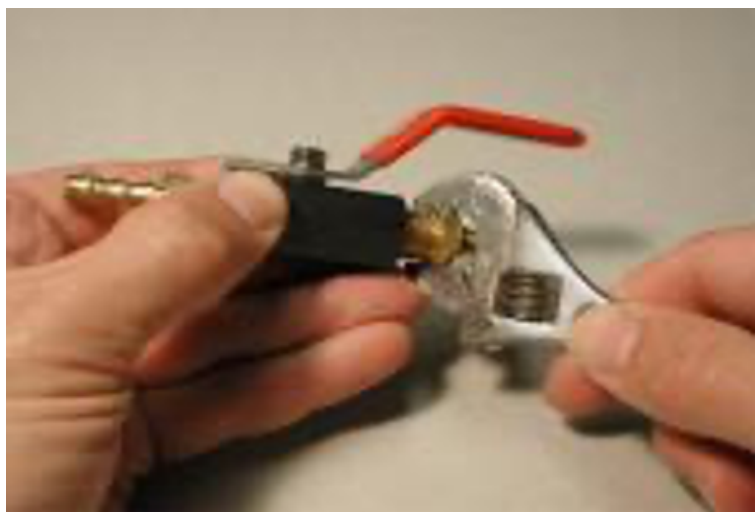
Installing the barb fittings on the ball valve.
