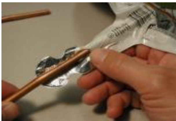
Inserting copper tubing
