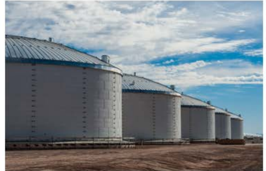
Molten salt storage tanks at the Solana Generating Station in Arizona, USA
